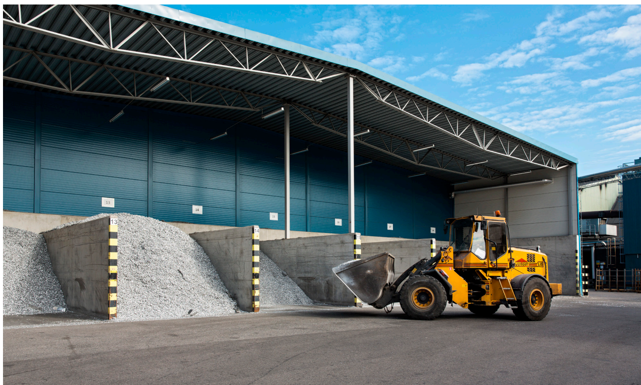
Recycling at the Finspång plant, Sweden.
