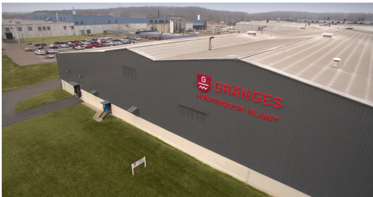
The Huntingdon plant in Tennessee, USA.
